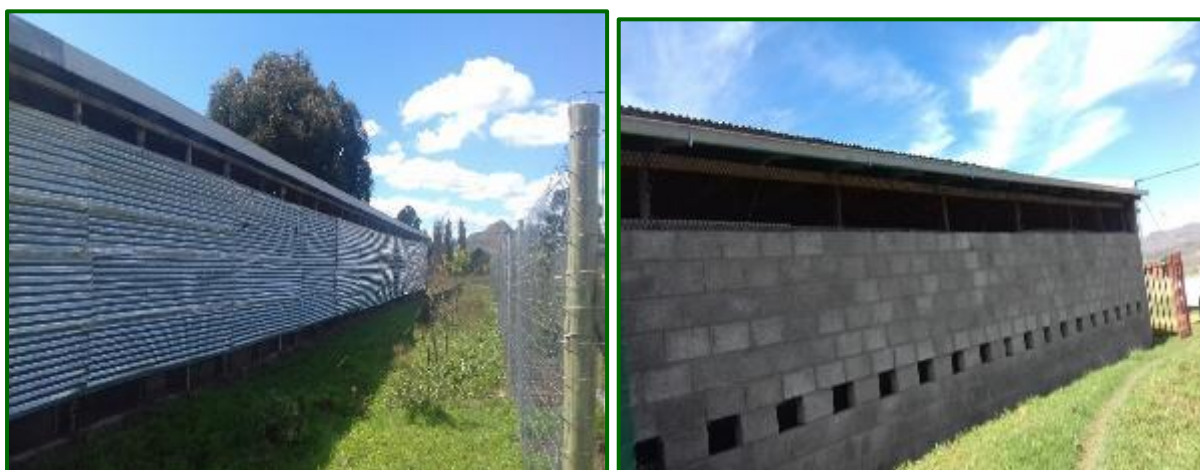
Figure 7: Layer houses with ventilation vents, birds and rodents excluders
