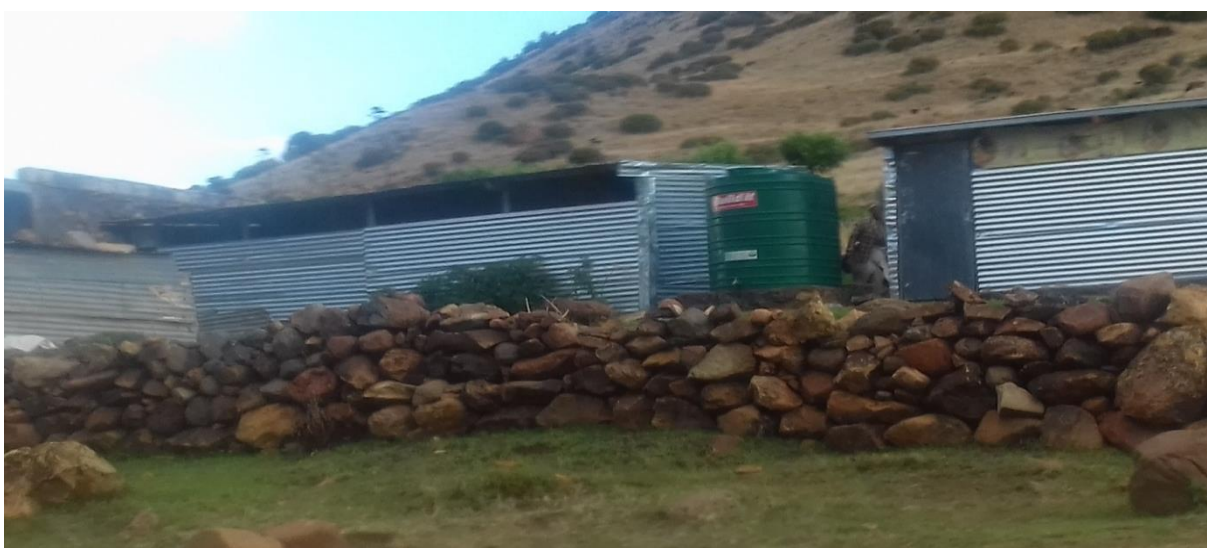
Figure 10: Housing infrastructure for young agripreneurs in Kolo RC in Mafeteng district
